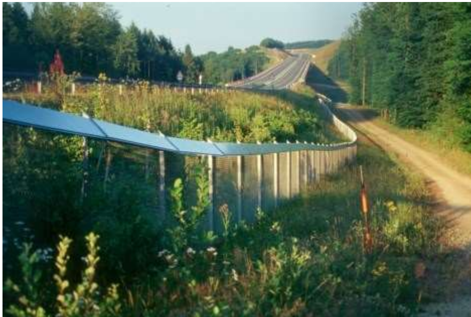
Figure 6: An der Autobahn A60 in der Eifel errichteter Wildkatzenschutzzaun - Wildcat fence built alongside the A60 motorway in the Eifel (Rhineland-Palatinate)
